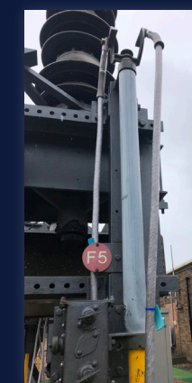
Substation Fixed Earthing
