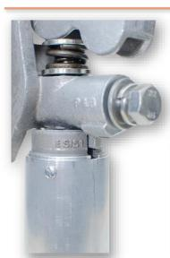
Clamp 'NIB' engages in the S9D socket to locate the clamp whilst being raised into position. The clamp does not require being fully opened/unscrewed as the socket controls the clamp whilst being fitted over the busbar.
